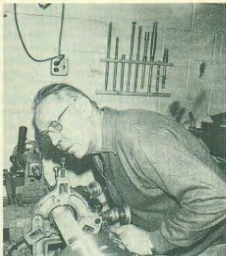
Ralph Stolle beginning work on a 2¼" x 2¼" aluminum blank.
